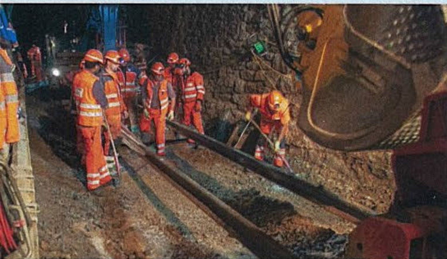
Track renewal means getting new ballast. Here track workers use shovels to help the Tyrex clear stone and debris until they reach the tunnel's floor.
